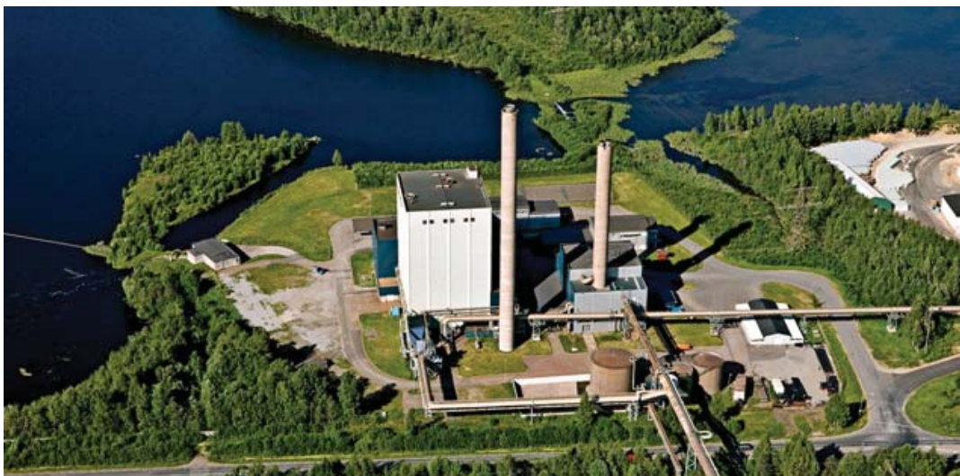
Figure 1.8 View over Luleå CHP, LUKAB, which supplies heat to Luleå
